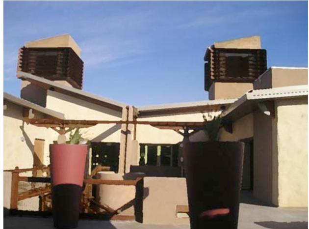
*Fig. 6: Downdraft evaporative cooling towers flank rainwater catchment, cascade and cistern at the Desert Living Center in Las Vegas*
