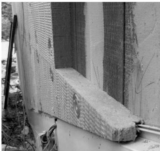
**Figure 3** Larkspur retrofit showing original redwood plywood siding sealed with mastic (air barrier) and 3 inches of new high-density mineral wool insulation.
