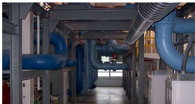
Effluent heat exchange facility at the main base Image courtesy of: Trane U.S., Inc.
