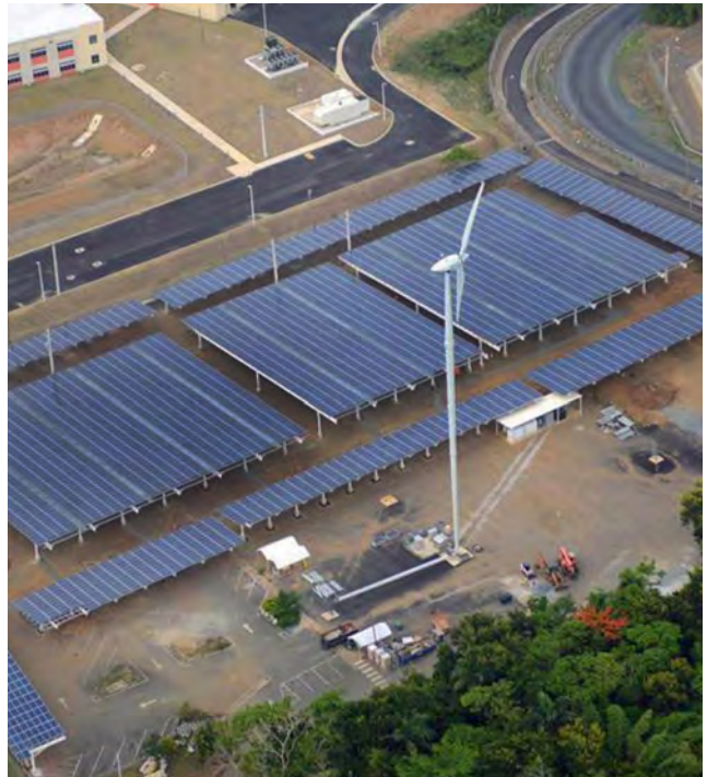
Parking lot PV canopy and neighboring wind turbine
